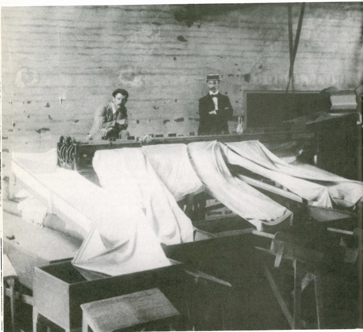
A Lemon Sizer (or Grader) installed as an experimental model in the Prenda Packing House of the Arlington Heights Fruit Co., 1899.
